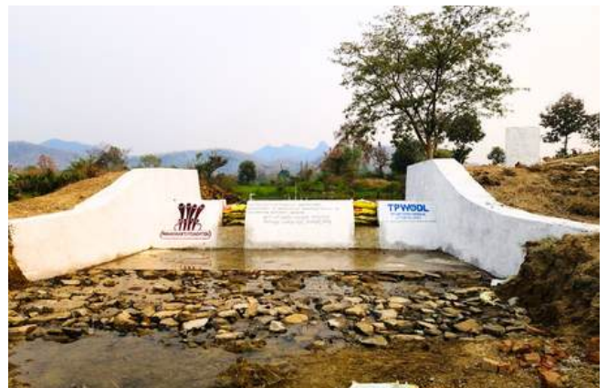
2 check dams and 4 drop structures have been constructed to enhance water resource management at M Rampur with the support of TPWODL.
